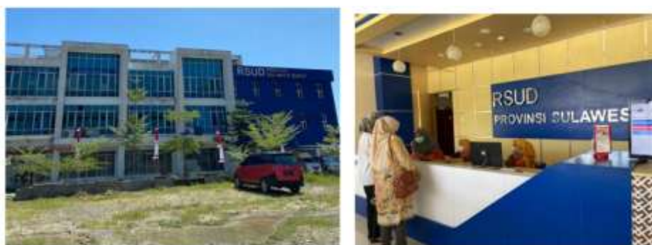
Figure 2. West Sulawesi Provincial General Hospital.
