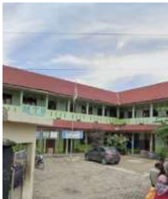
Gambar 3. Madrasah Tsanawiyah Laboratorium Jambi.
